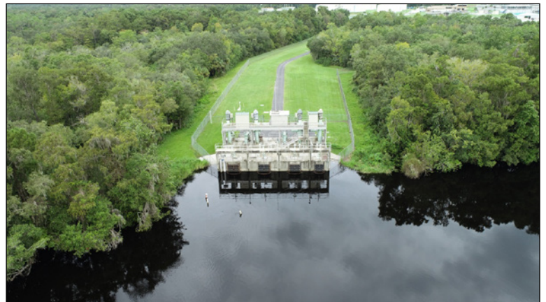
Figure 2. Existing intake on the Peace River. (photo: Peace River Manasota Regional Water Supply Authority)
